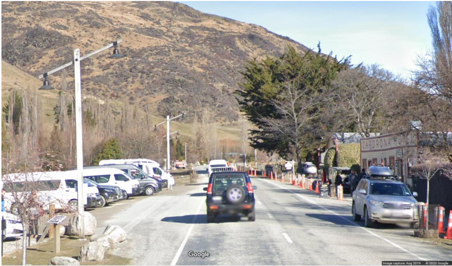
Cardona Valley Road Street Light Poles
