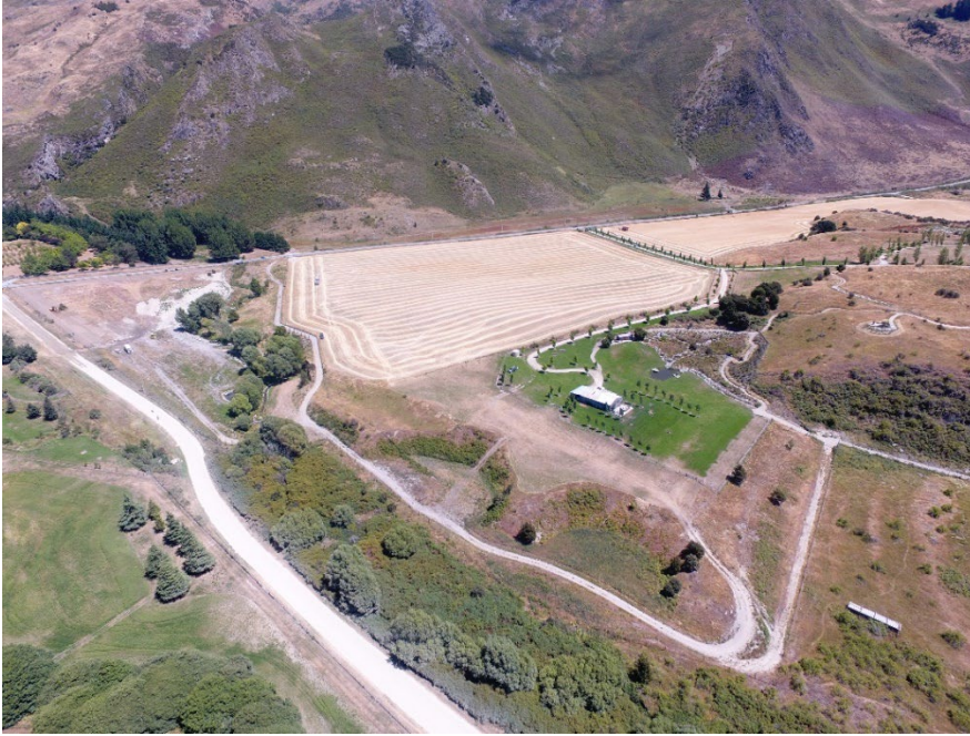
Drone image of the surrounding site, with the existing woolshed centre right of picture. (23 Jan 2023).
