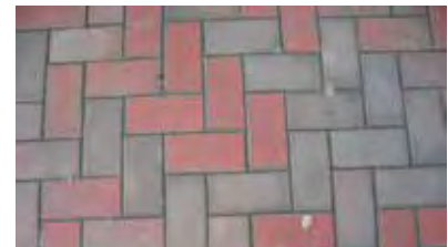
Avoid modern coloured tiles, which are inappropriate to historic character.
