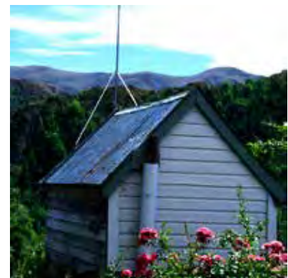
Small shed-out building.
