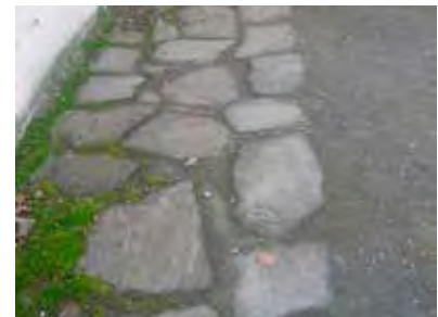
Encourage stone detailing set in crusher dust and gravel pathways.
