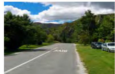
Narrow carriageway gravel shoulders, grass swales and verges with street trees.
