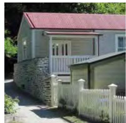
The simple shed form used to the rear of the Postmaster's Restaurant.
