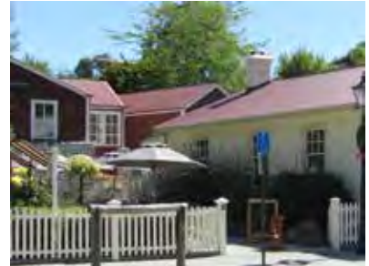
New development to the rear of the Postmaster Restaurant, viewed from eastern end of Buckingham Street, reflects contemporary two storey development incorporating simple shed forms in a grouped arrangement of buildings.
