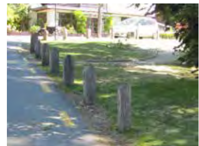
Good example of simple timber bollard.
