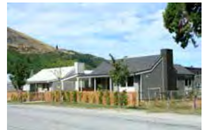
Example of recent medium density residential development in Arrowtown, with a single house still facing street frontage on each lot.
