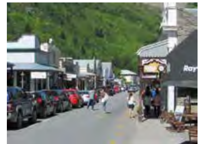
Western end of Buckingham Street showing the narrow nature of footpaths, verandas and positioning of buildings against front road boundary.
