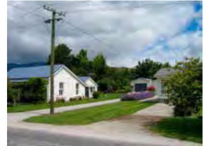
Garage set to rear of section.
