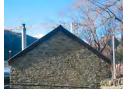
The simple form of the shed.
