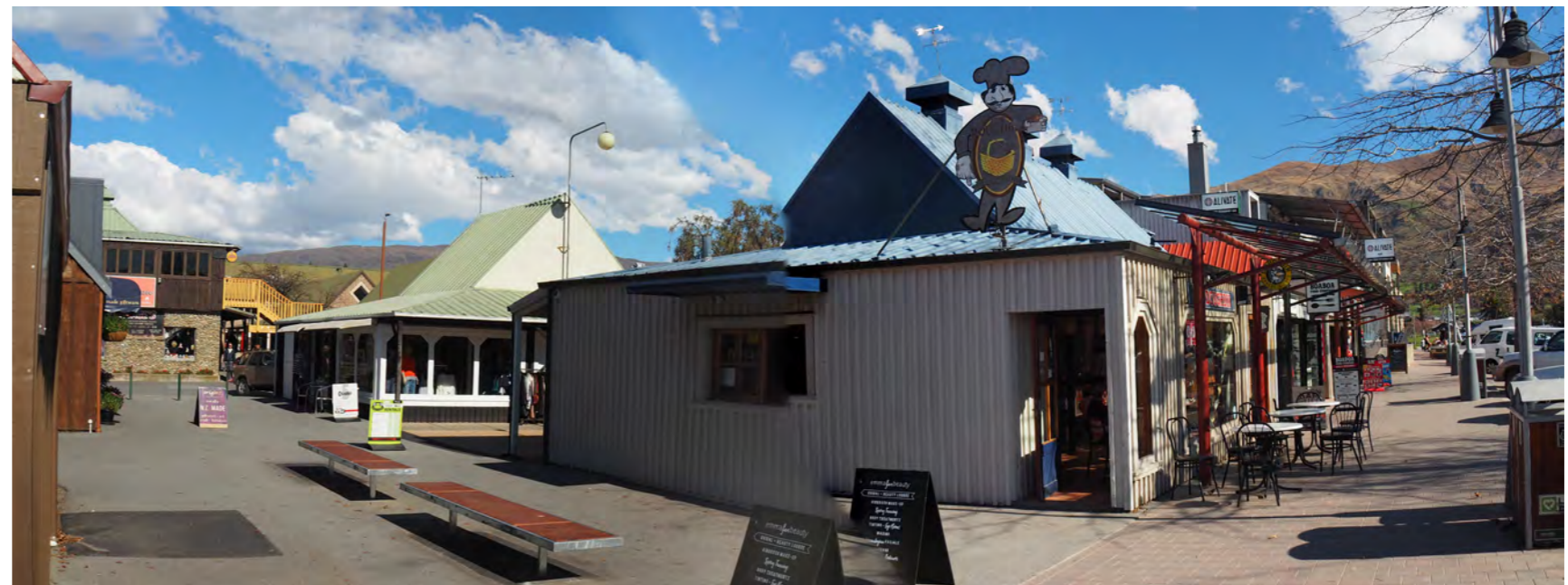
Existing low rise buildings and publicly accessible lane network
