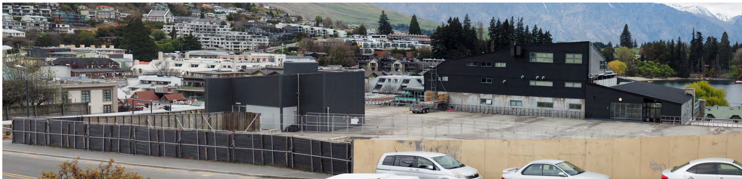
Elevated view of Man Street Car park (West) from 33 Man Street (first floor)
