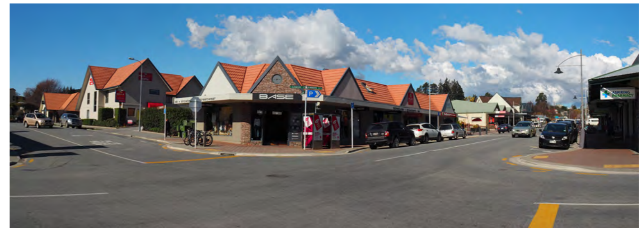
View South East towards the corner of Helwick and Dunmore Streets
