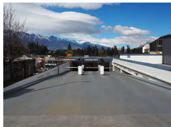
Existing Man Street Car Park ramp/ (Eastern View Shaft)
