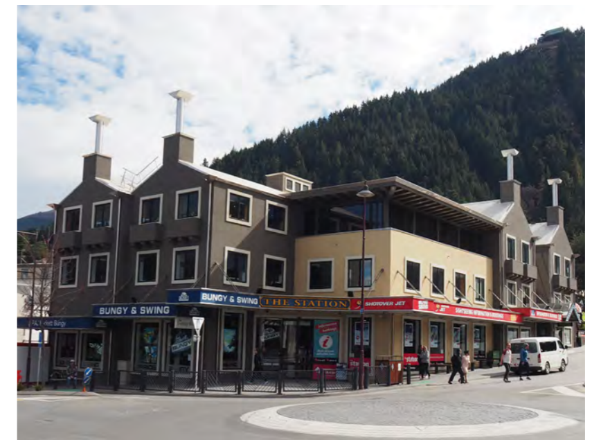
The Station Building (rear, excluding chimneys), Duke
