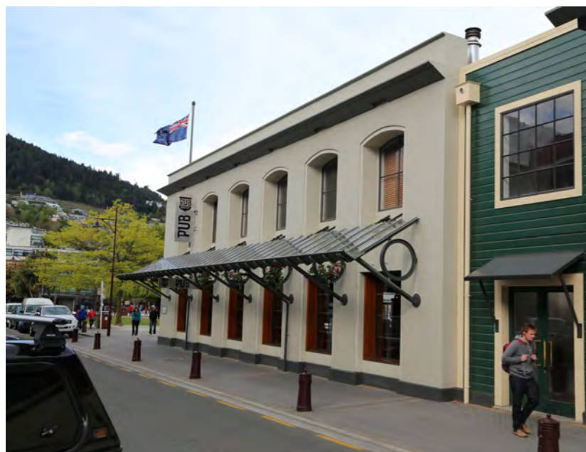
Steamer Wharf, Beach Street
