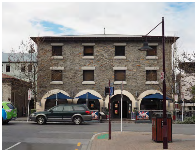
Ngai Tahu Courthouse Development, Ballarat Street
