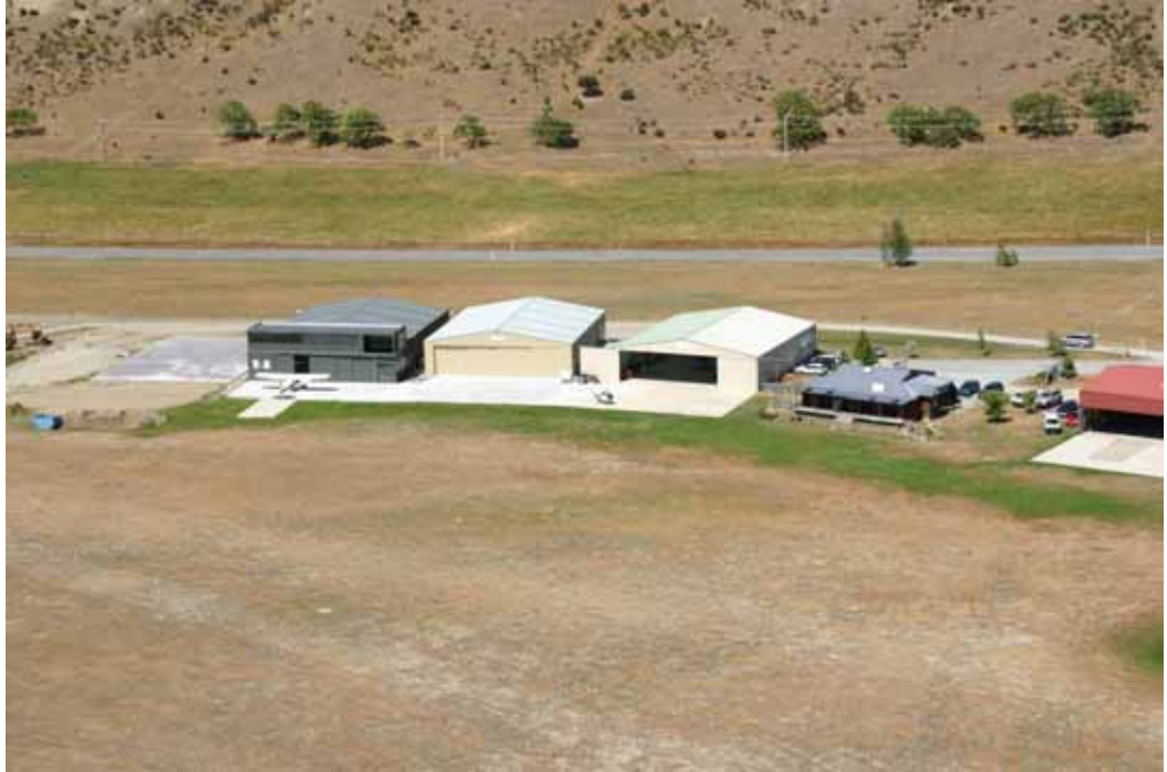
Figure 7-7: Hangars in the Helicopter Zone with existing concrete TALO areas in foreground. The proposed helicopter clearway extends out across the grass to the runway. Note irrigated apron verge to eliminate dust hazard.
