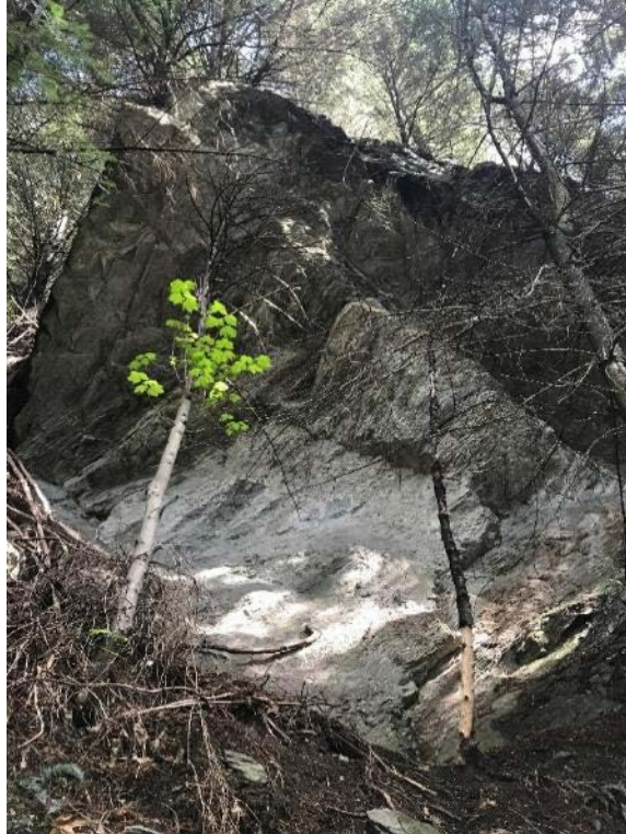
Figure E 37 - Photograph looking up at cliff present between Brewery and Reavers Creek. A loose block is present at the intersection of two joint sets. Photograph taken looking upslope towards the west (45.11414; 168.391672; 580m asl).
