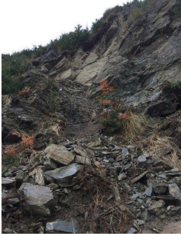
Figure E 11 - Close-up photograph of recent scarp and rockfall debris on outcrop present on ridgeline looking west and shown in Figure E10 (45.042570 168.385761; 985m asl).
