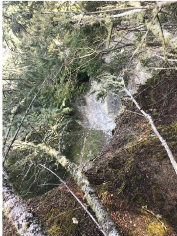
Figure E 29 - Photograph looking towards cliff above boulder the field in the channel. Cliff outcrops along ridgeline next to the Skyline Gondola and is approximately 20-50m high (45.124640; 168.385355; 735m asl).
