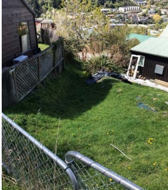
Figure E 22 - Photograph of small channel through residential properties directly above culvert intake. Taken looking east (45.126229; 168.391439; 365m asl).
