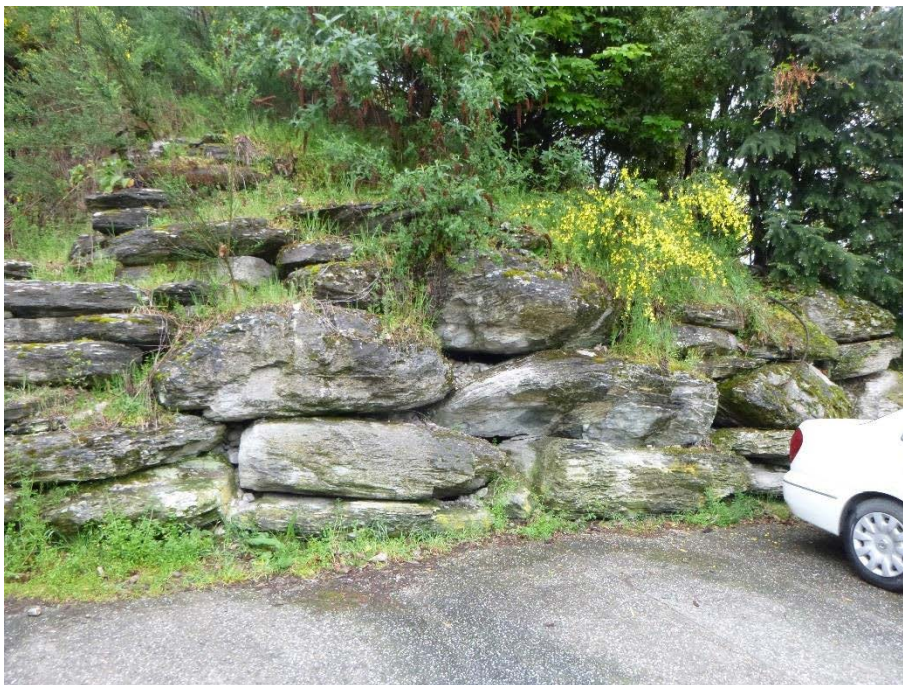
Figure 11 - Numerous boulders used to construct informal retaining wall on the surface of Reavers Fan (2018)
