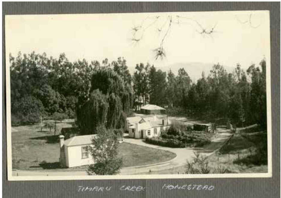
The Timaru Creek homestead went below the lake after 1958
