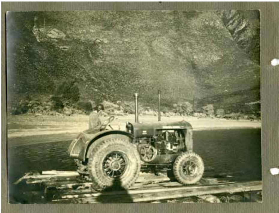
Transporting the tractor up the lake by barge
