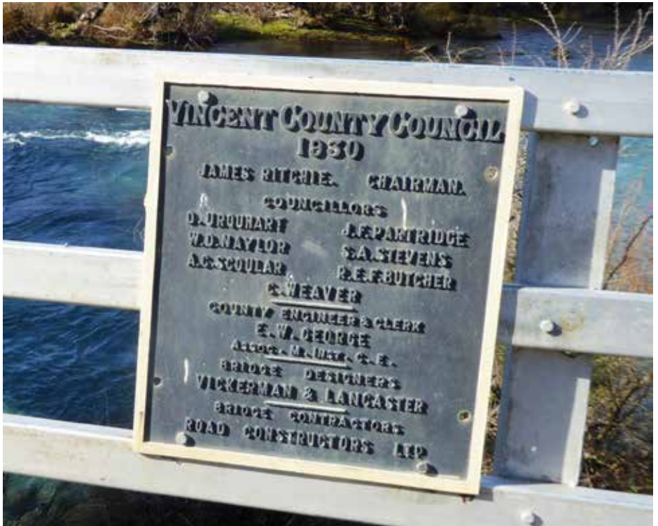
Plaque, Camphill Road Bridge, showing the opening date as 1930 Photograph, Trevor Chinn
