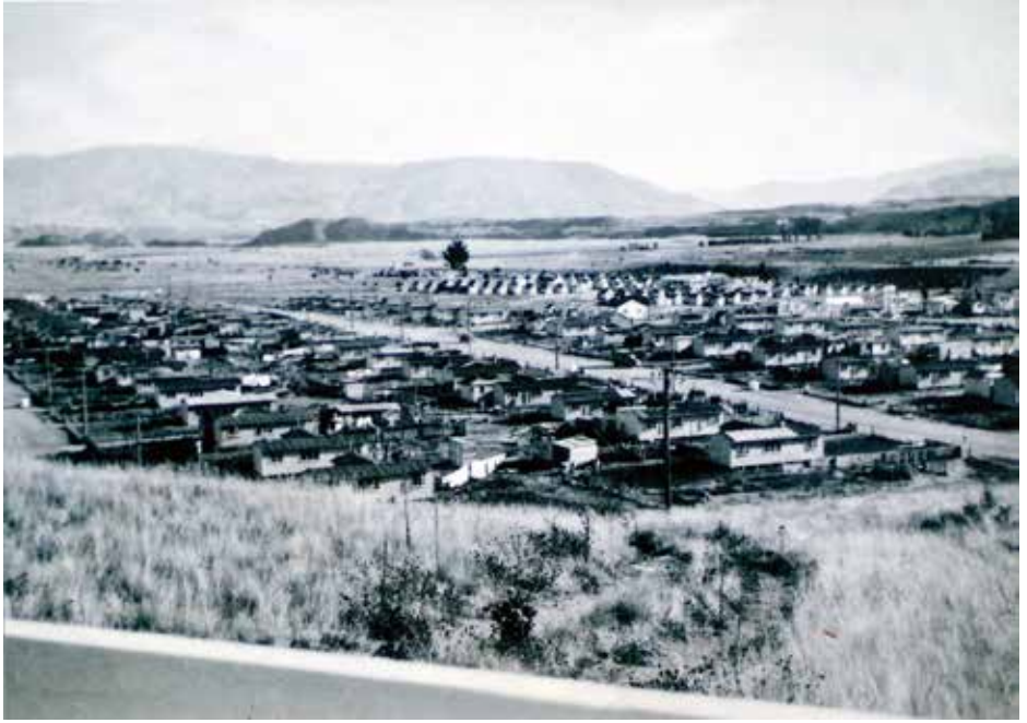
MOW Camp at Timsfield during the building of the Dam
