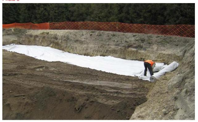
Mixed soils depository and placement of geotextile fabric as visual indicator (Courtesy of Golder Associates validation report December 2008)
