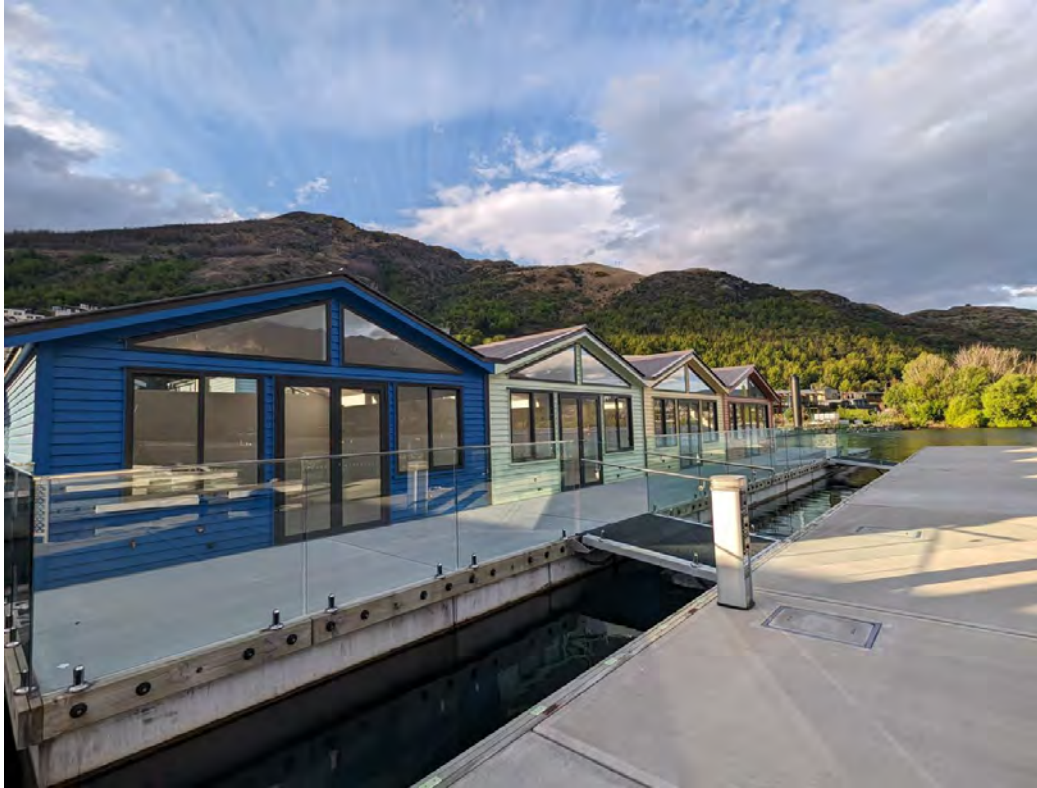
Figure 2.2 – Four eastern-most floating buildings
