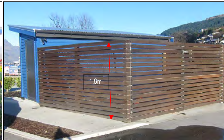
East elevation and fence
