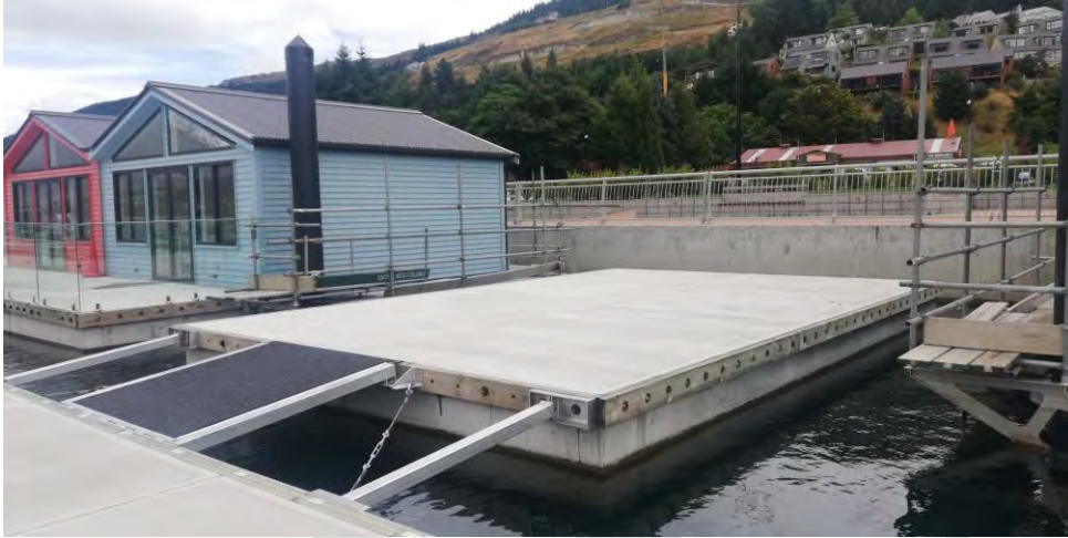
Figure 3.1 – Floating pontoon to the east of the floating buildings
