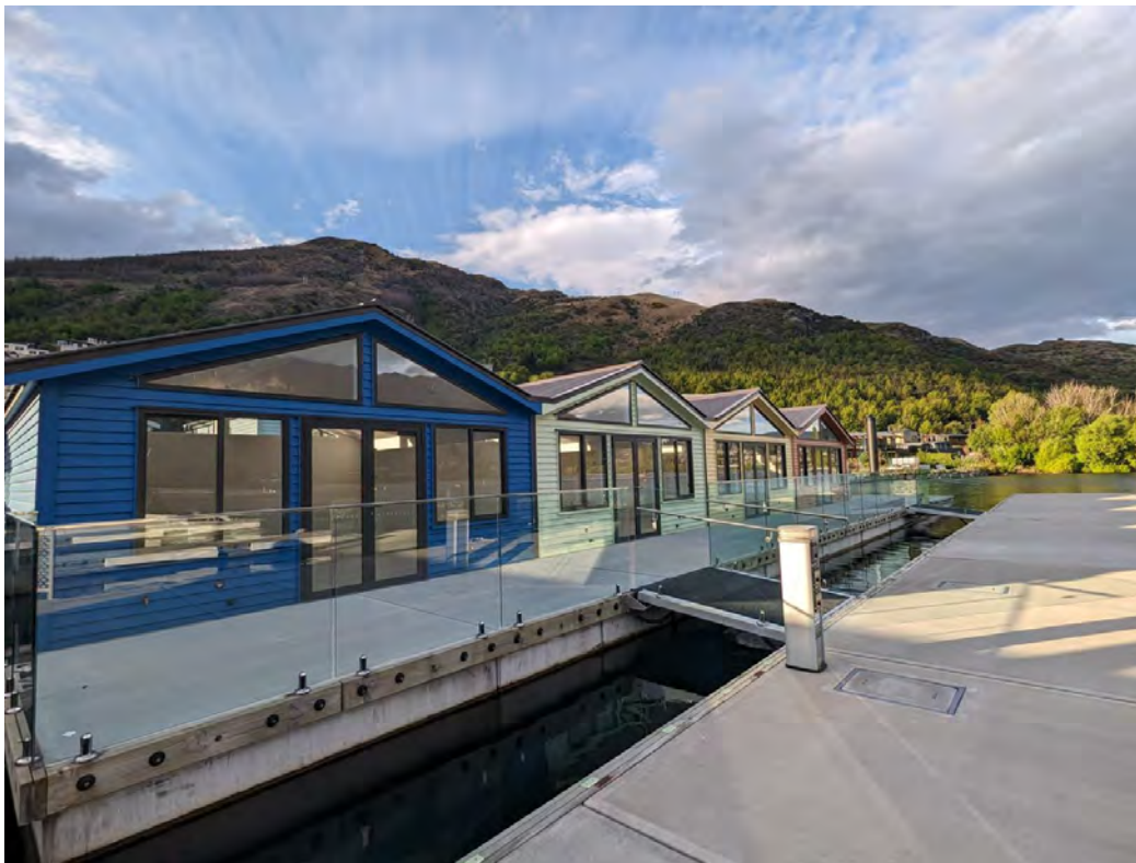
Figure 1.3 – Four eastern-most floating buildings
