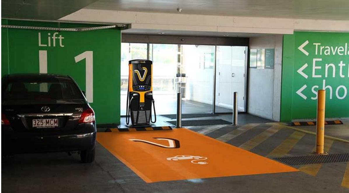
At 165kg it is one of the lightest units available, reducing installation complexity and allowing for easy relocation if necessary. Despite its size and weight, it is rated to deliver 50kW continuous DC output. At full power it requires 55kVA of transformer capacity (ie 80A @ 400V). The unit is 2m tall and 0.7m wide (about the size of a door) and approximately 300mm thick. As can be seen in the image (Kaiwaka, north of Auckland), they are relatively attractive units:
