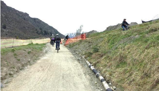
Figure 18: Steep gradients and loose surfacing between Frankton and the Shotover River
