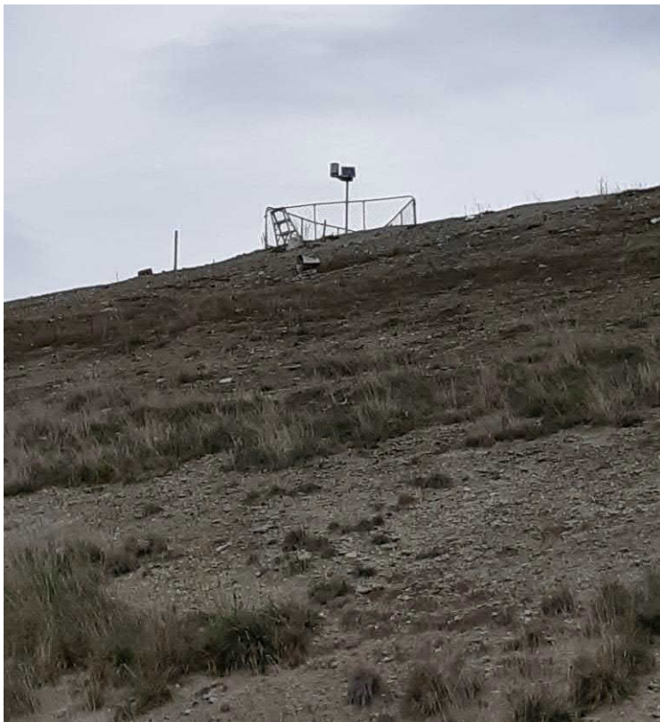
Figure 1: Existing batter on completed landfill area
