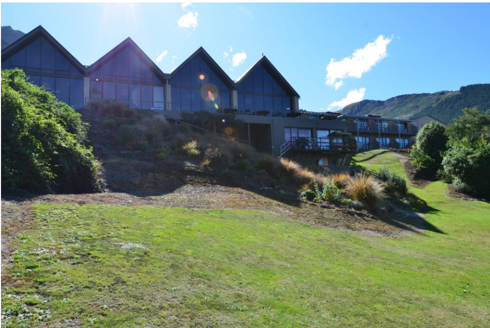
View of the conference facilities and restaurant at the Aspen Hotel.
