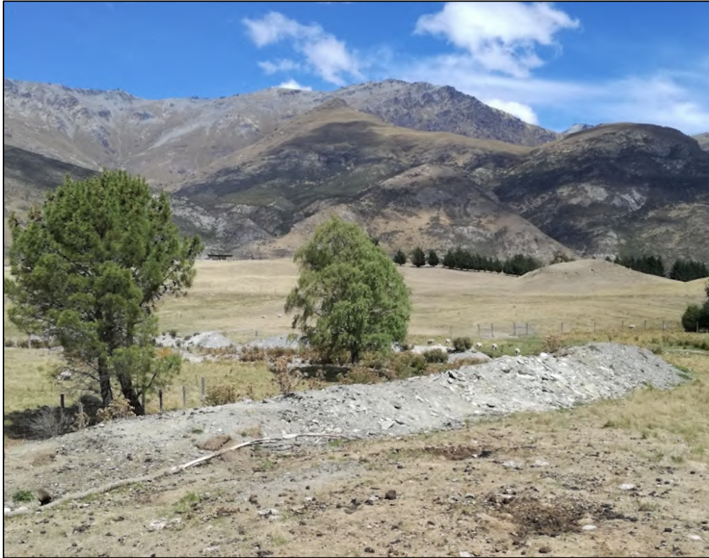
Figure 4.1.1: Excavated Spoil Material Next to Race
