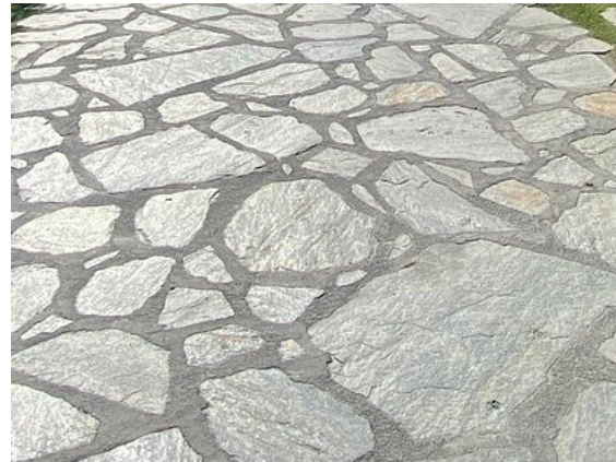
P1 a Natural blue stone schist paving, used as both smooth textures and textured/honed
