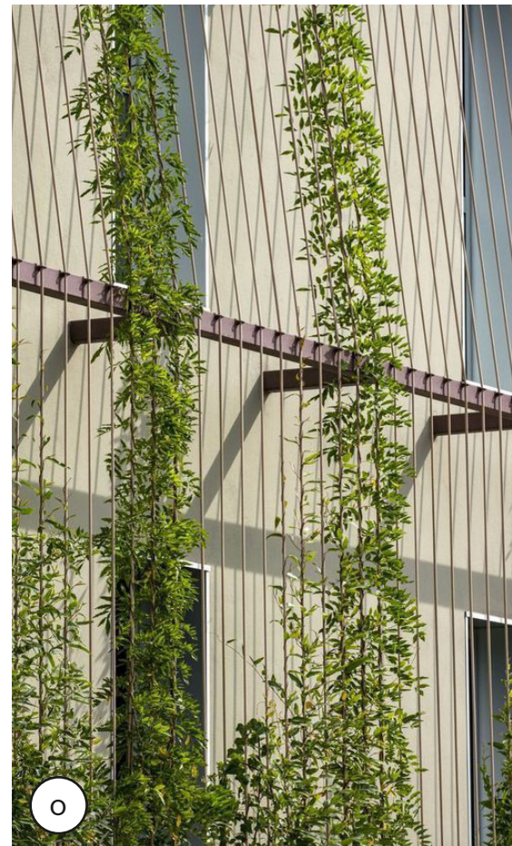
Laneways - Vertical vegetated rain chain wall, celebrating rain water through visual means
