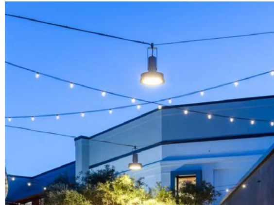
L3 Overhead festoon lighting
