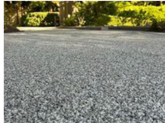
P4 Permeable Resin Bonded Gravel
