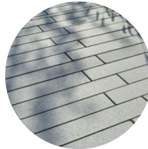
P2 Linear Feature Paving - Non-Permeable
