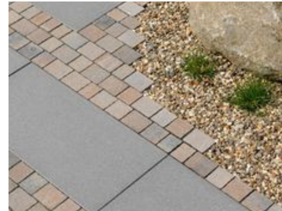
P3 Paving Setts to building trim, integrated into P2 linear feature paving
