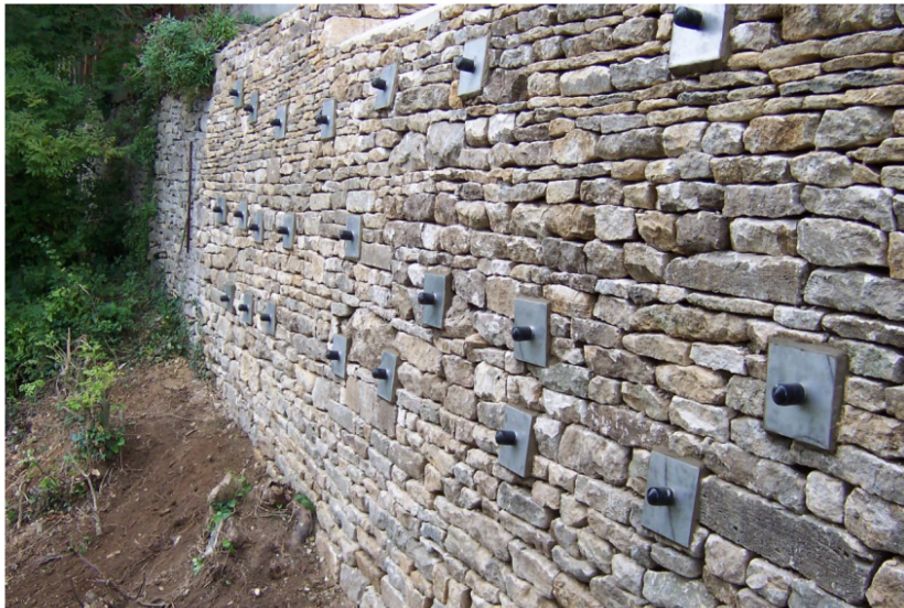
Figure 3 – Closely spaced self-drilling anchors with small plates
