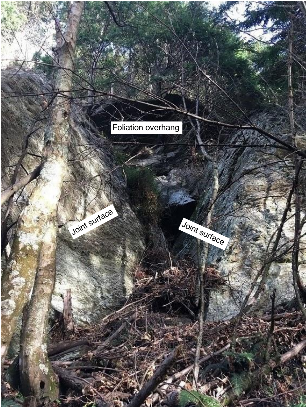
Photograph 17b. DL2 map area general photograph. Historic post glacial wedge failure in schist bluff.
