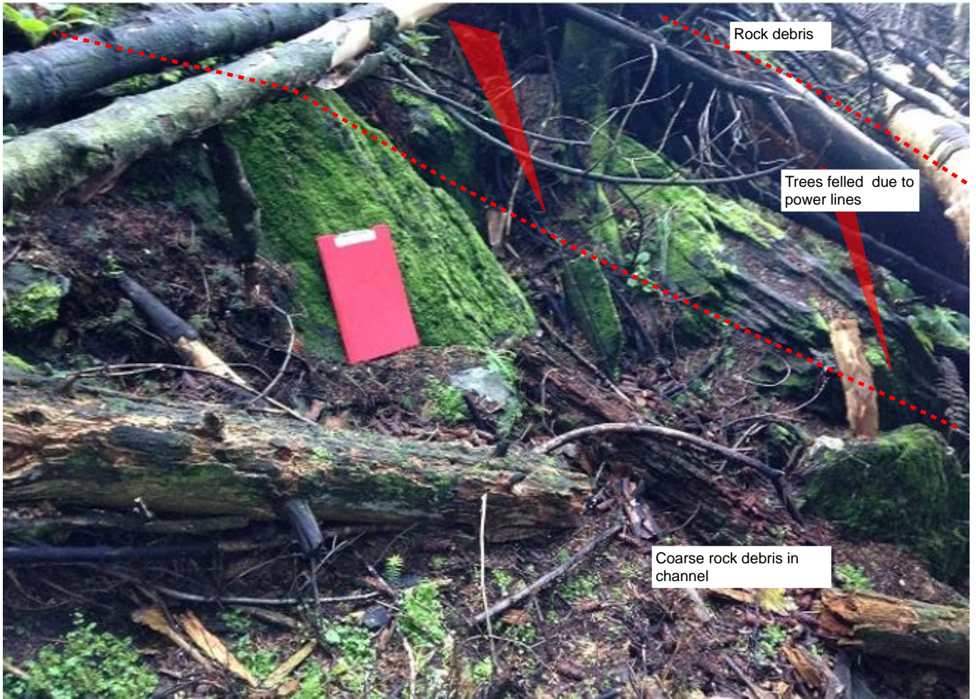
Photograph 14a. Flow channel Section 11a.
