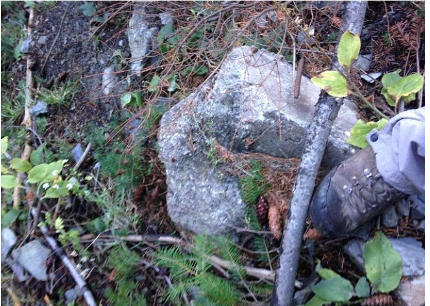
Photograph 28a. Concrete indicating the presence of fill materials
