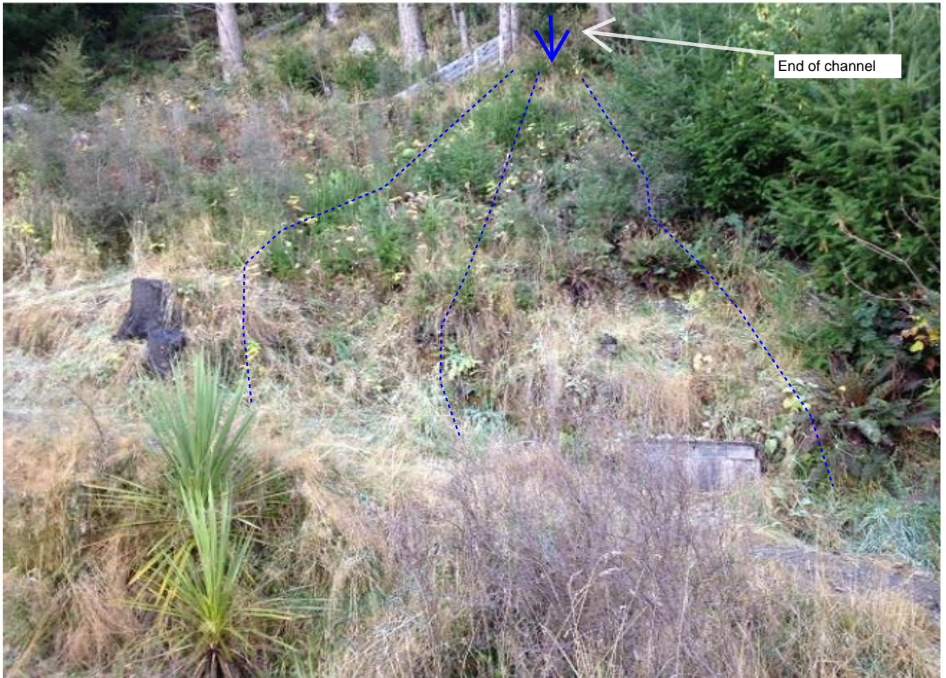
Photograph 11a. Slope area immediately below the defined DL1 channel. Vegetated slopes no clear scour/erosion or active down slope movement of materials. Very dense vegetation comprising young pines on the left of the photograph.
