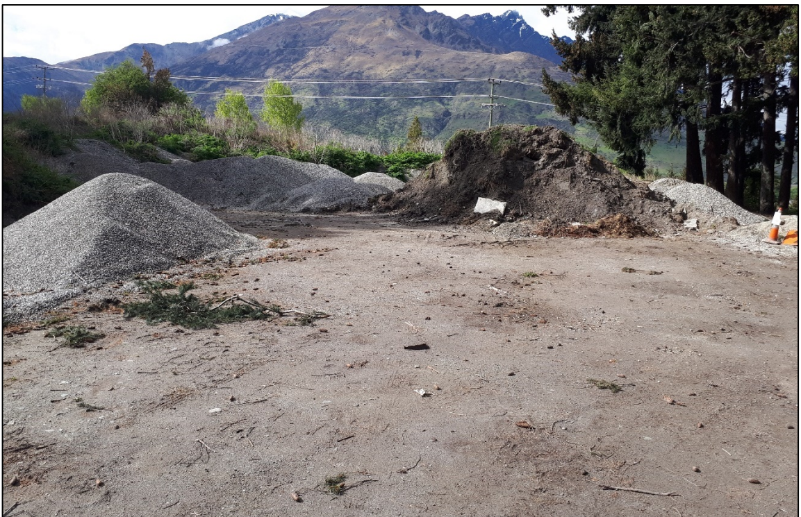
Figure 17: Stockpiles of material within Sec 159 Blk III Shotover SD.
