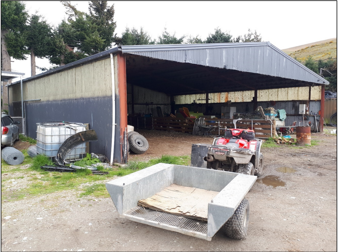
Figure 11: Former hanger building at 28 Strains Road.
