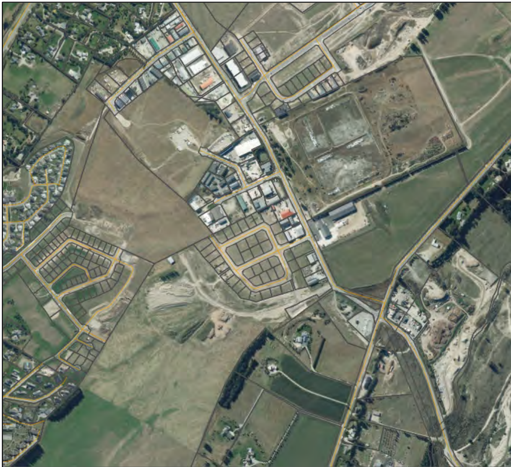
Figure 3: Aerial Photography of the “Wanaka Industrial Area” (Source: QLDC website, photography from 2019)
