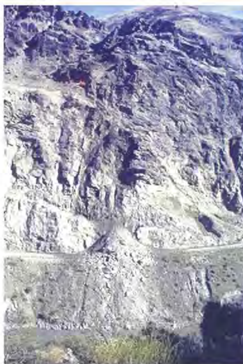
Photograph 3 - Rock Slope Failure at Nevis Bluff, along State Highway 6
