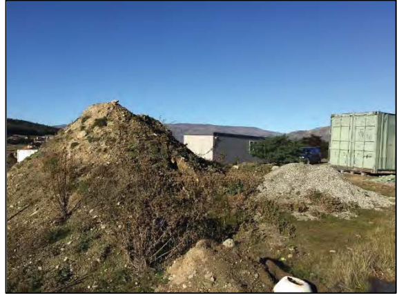
Plate 4: Gravel and earth stockpiles east of groundworks yard
