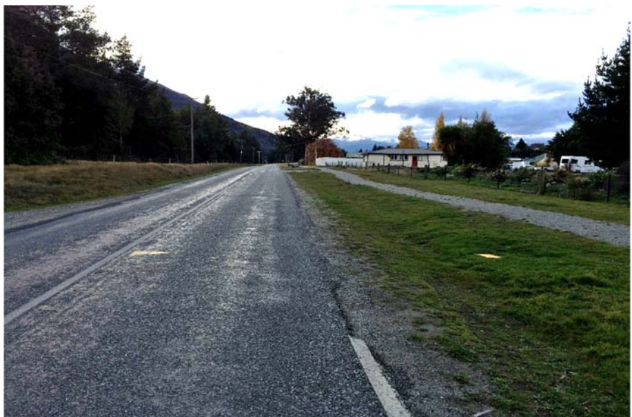
Photograph 3: Domain Road (North of Cemetery Road) Looking North
