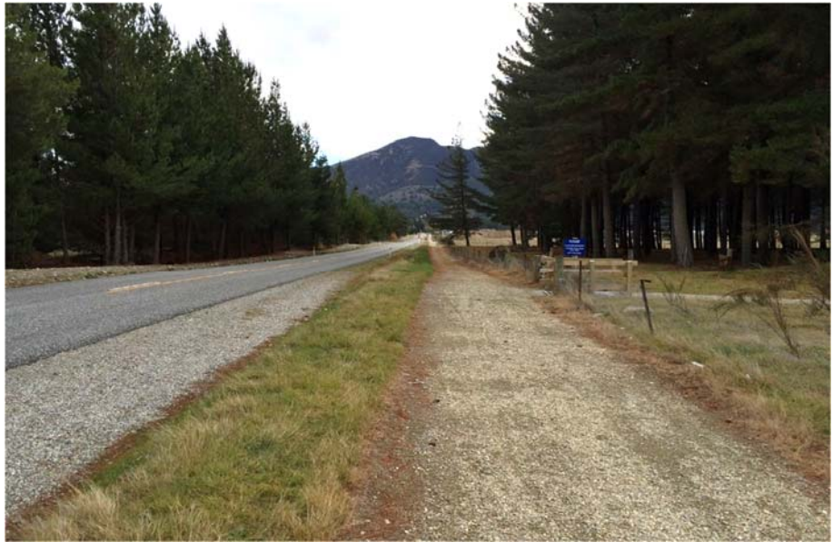
Photograph 8: Cemetery Road Footpath/Cyclepath, Looking West
