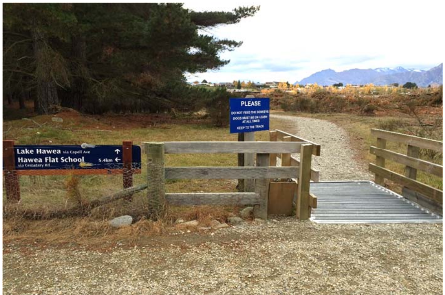
Photograph 10: Capell Avenue Footpath/Cyclepath, At Cemetery Road
