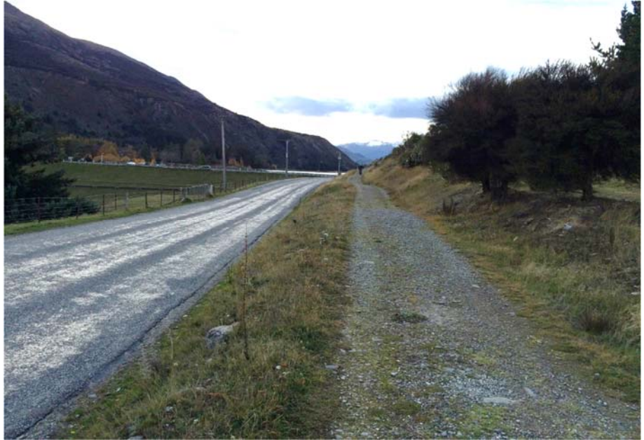
Photograph 9: Elevated Footpath/Cyclepath on Eastern Side of Domain Road (North of Cemetery Road)
