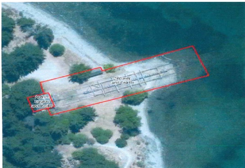
3a and 3b - Antrim Engine and Boiler, and Slipway and Cradle, Kelvin Peninsula. The Extent of Place is shown by the red outline
