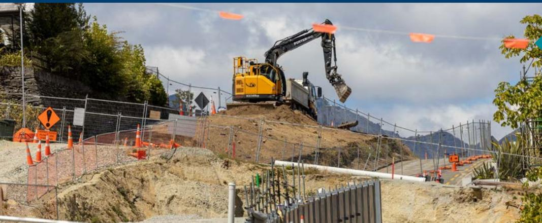
A digger works on constructing the new link between Melbourne and Henry Streets. In the foreground you can see the large steel sheets which have been dug into the ground to help form the new road.
