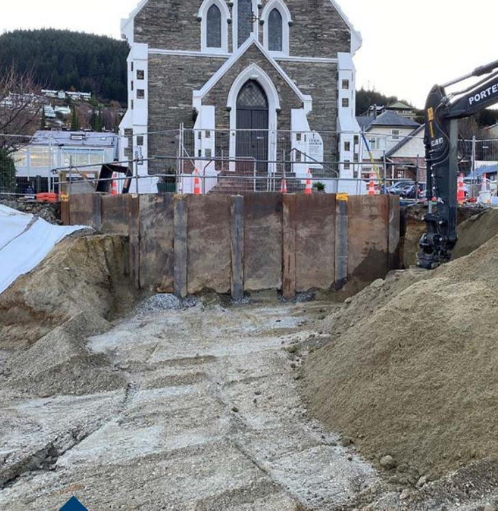
A steel wall is being built in front of the St Joseph's church and school, ahead of the main retaining wall construction.
