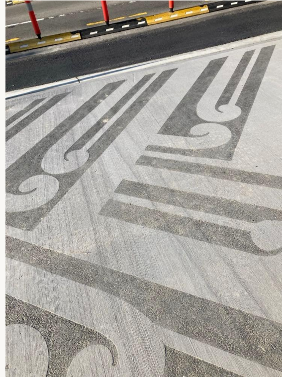
Vapour blasted concrete – Pipitea Marae - Wgtn
