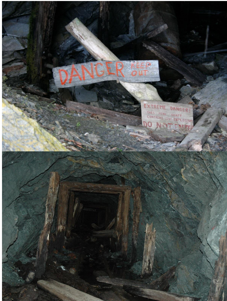
Figure 3 – Existing mine entrance that can be made safe,
