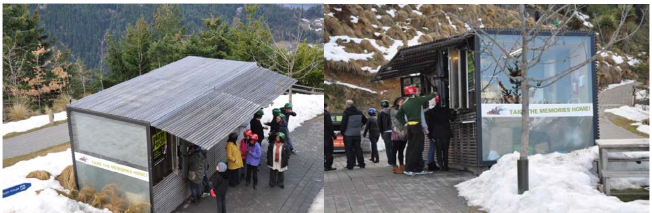
Photos 3. & 4. Illustrating the Photo Kiosk Building on Site as Approved by RM070488
