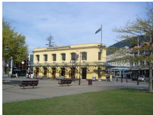
Steamer Wharf, 88 Beach Street
