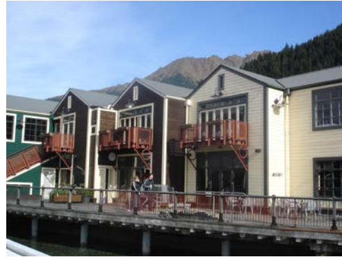
Steamer Wharf, 88 Beach Street
