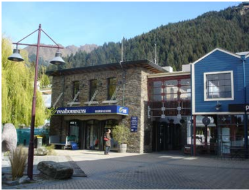
Steamer Wharf, 88 Beach Street
