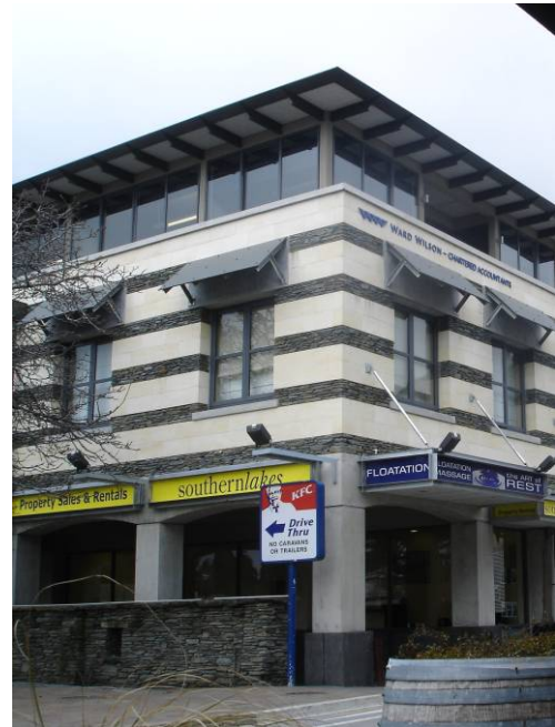
Ward Wilson Building, 10 Athol Street
