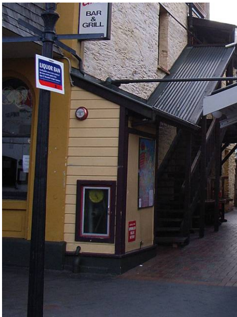
19, Ballarat St (painted weatherboards)
