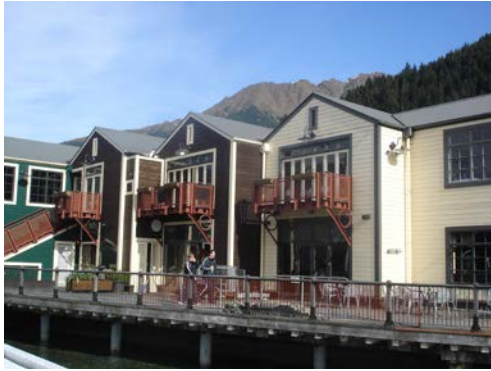
Steamer Wharf, 88 Beach Street
