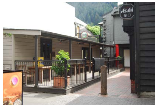
Pedestrian Arcade from Searle Lane to Mall
