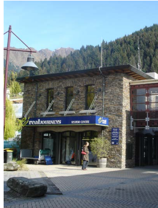
Steamer Wharf, 88 Beach Street
