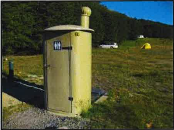
Self contained toilet
