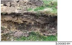
Excavation measures ~3 m x 1.5 m. Bedrock and groundwater was not encountered
