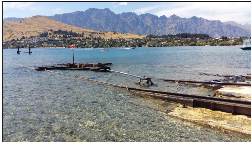
Figure 4 Photo showing the slipway 'cradle'
