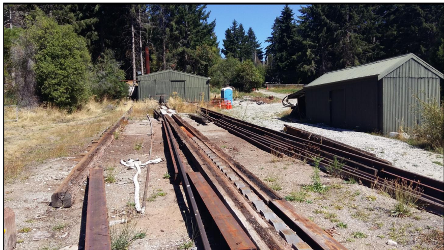
Figure 5 Photo showing slipway and associated buildings (Antrim Engine located in the shed in centre of picture – chimney visible)
