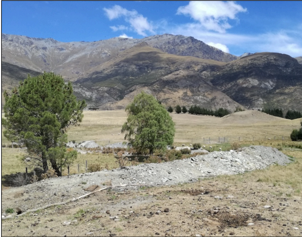
Figure 4.1.1: Excavated Spoil Material Next to Race
