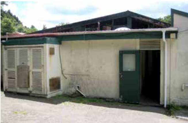
Example of unlit rear of a bar
