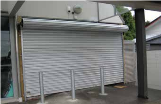
Example of roller shutters
