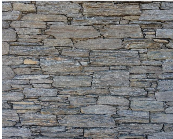
Fig 1: Dry-stacked schist
