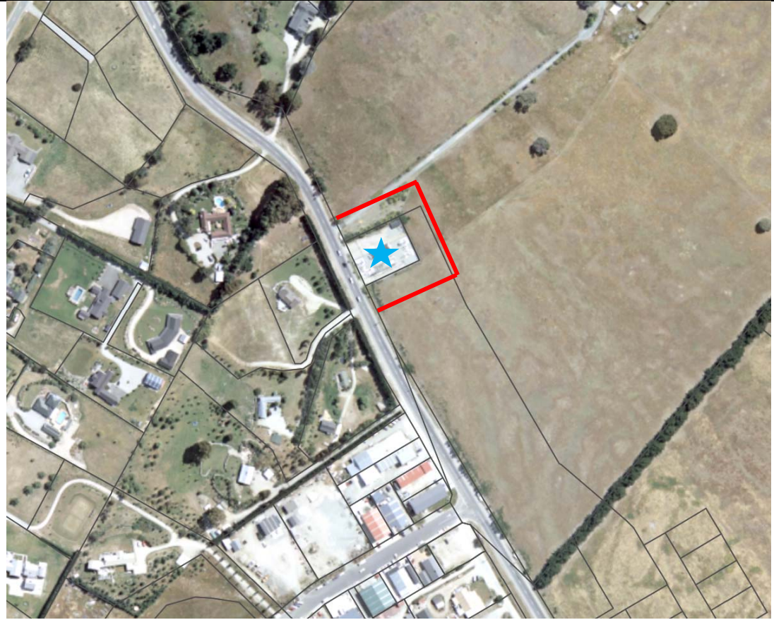
Figure. 1 Aerial photo of subject site showing location of Aurora substation (blue star) and surrounding land approximated by red border which is approximately 20m from the boundary of the Aurora site
