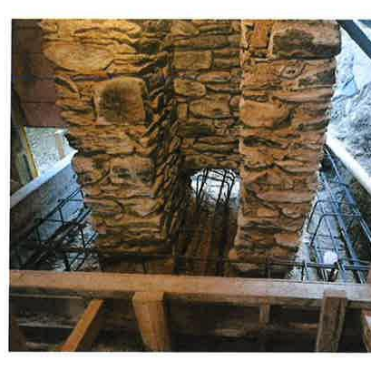
2023 concrete slab foundation ready for pouring
