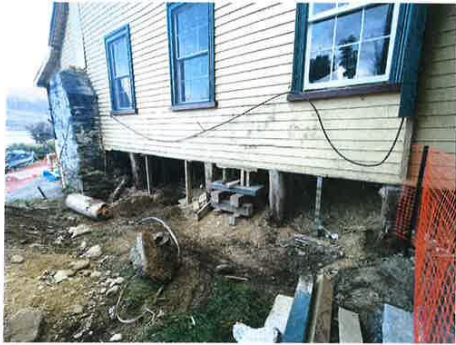
N Elevation preparation for new piles
