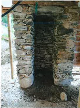
Original 1870 chimney Foundation (Large rocks!)
