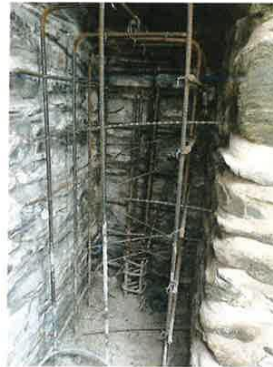
Reinforcing cage and ties for concrete
