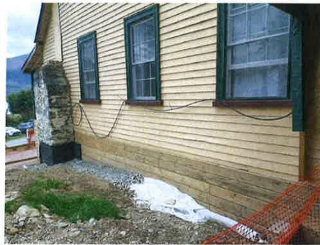
Substantial timbering for seismic bracing
