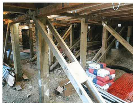
2023 piles with substantially engineered bracing
