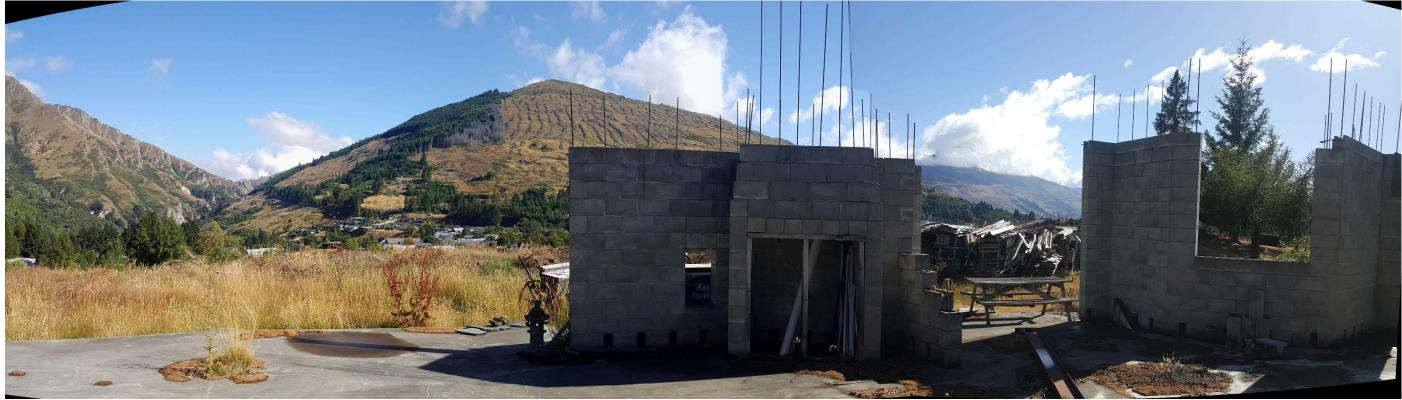
Photograph A: Taken standing on the northeastern corner of the building platform on proposed Lot 41. The walls and floor pad of the partially built dwelling (RM980348) extend approximately 8m to the north of the northern edge of the building platform. The upper edge of the escarpment is approximately 20m to the north of the northern edge of the platform.
