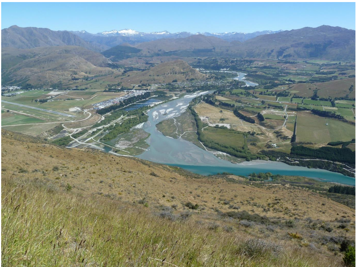
Plate 8: View over the Kimi-akua / Shotover Delta; Willows have been removed from upstream of the confluence, the flood retention wall was constructed in 2011. D Palmer, 21 January 2013.
