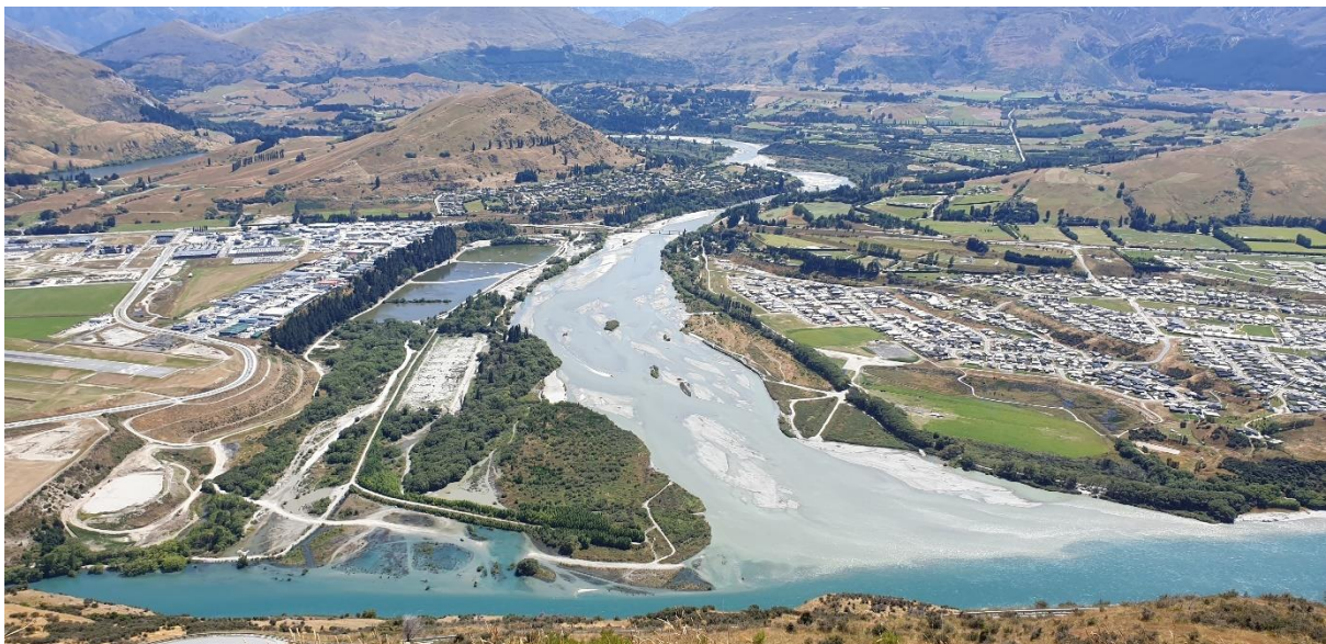
Plate 10: Shotover Disposal field installed; infilling of Shotover Country. A broad portion of the flood plain vulnerable to inundation. A high flow of about 450 cumecs occurred in the first week of February 2020. D Palmer 7 February 2020, D Palmer
