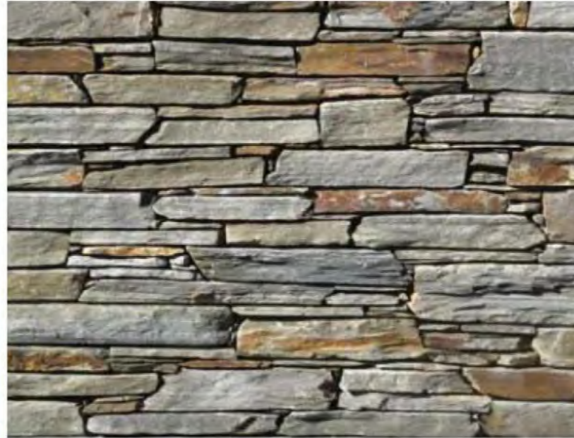
4 Stacked stone cladding
