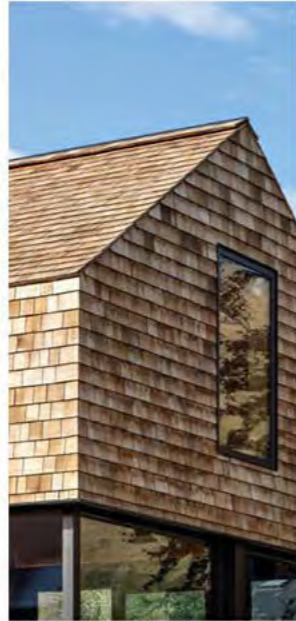
2 Timber shingle roofing
