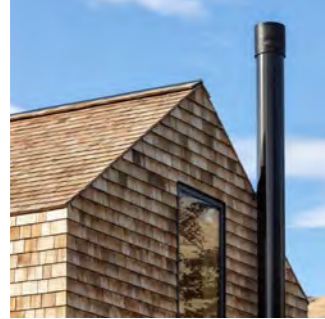
Timber shingle roofing & cladding_
