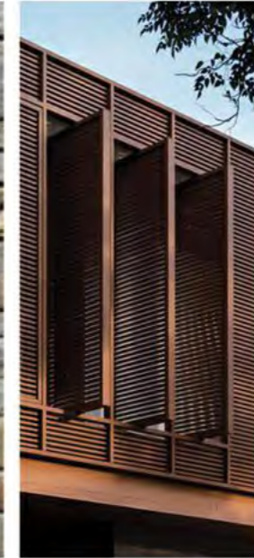
5 Operable timber louvres
