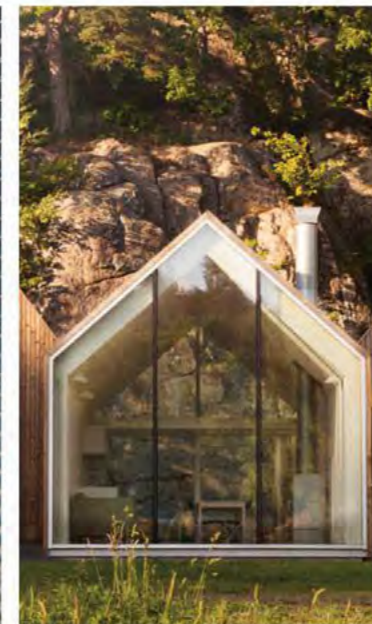
9 Black powdercoated aluminium joinery
