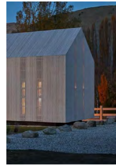
19 Timber rainscreen cladding
