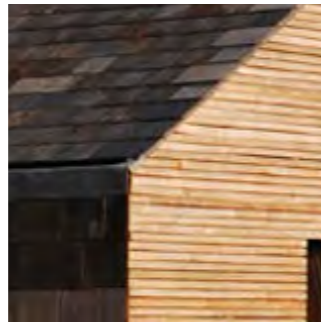
Timber shingle roofing w concealed gutter_
