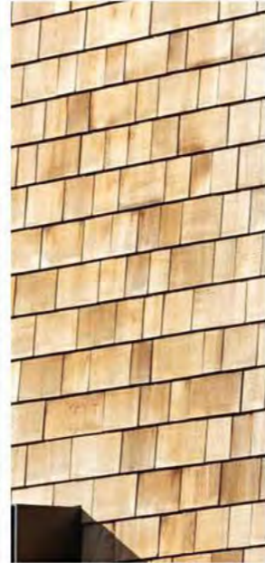
3 Timber shingle cladding
