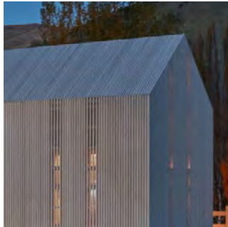
Timber rainscreen cladding_
