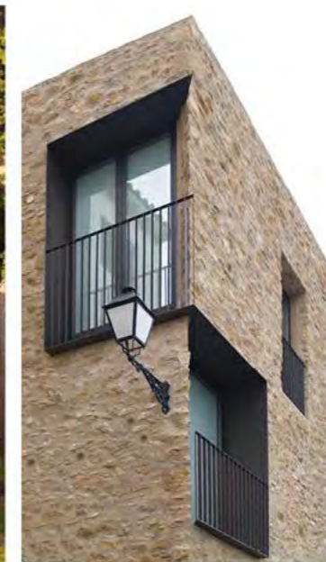
10 Chamfered steel plate reveal
