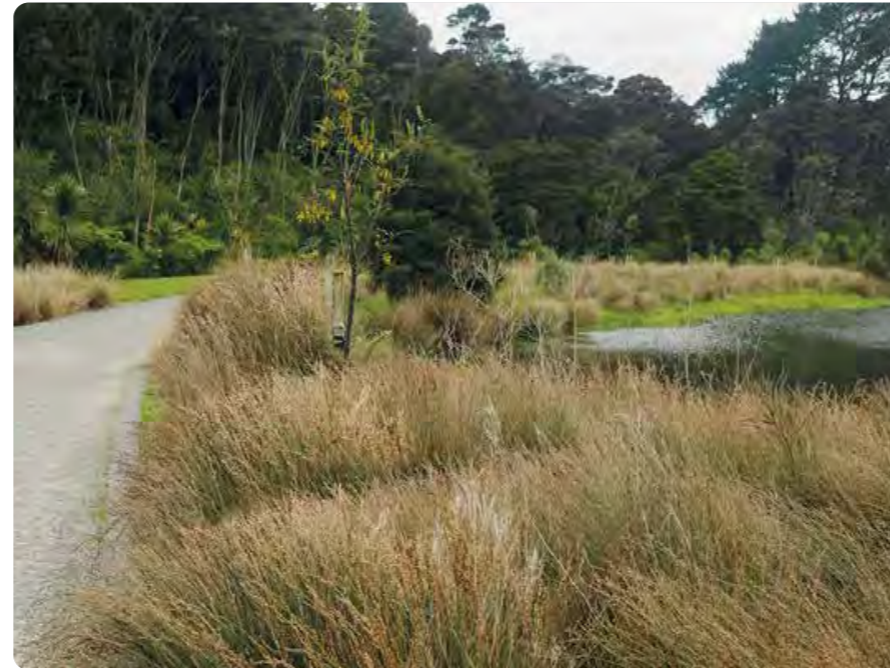
Stormwater wetland with native planting and walking paths.
