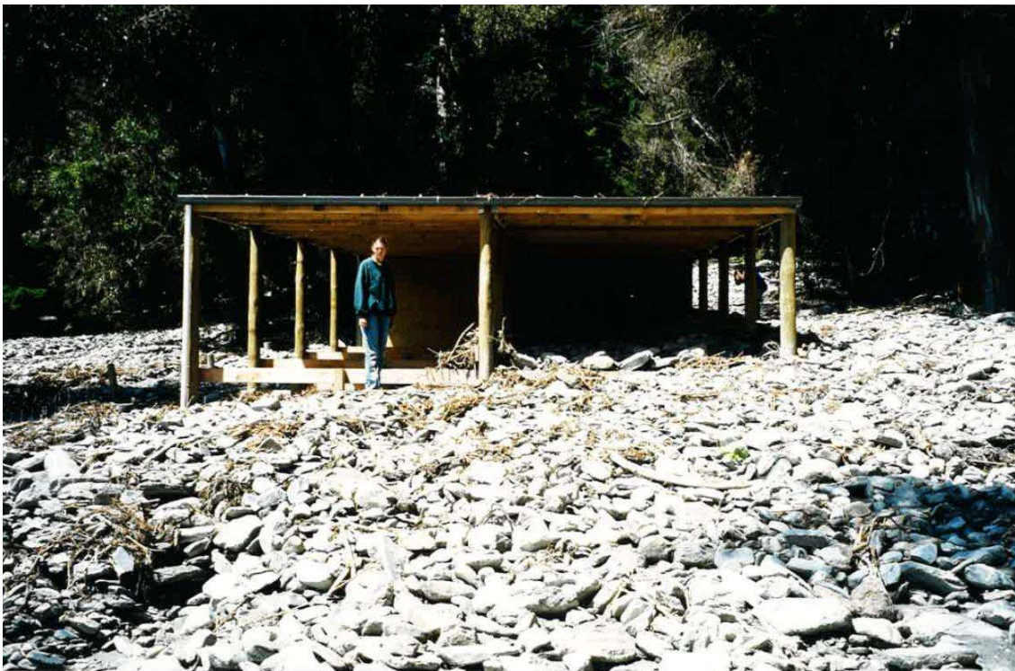
Photograph A3: Deposition of boulder gravel on the Stables Fan following the 1999 debris flow. The building is the old stables that was inundated by about 1.5 m and was subsequently abandoned.
