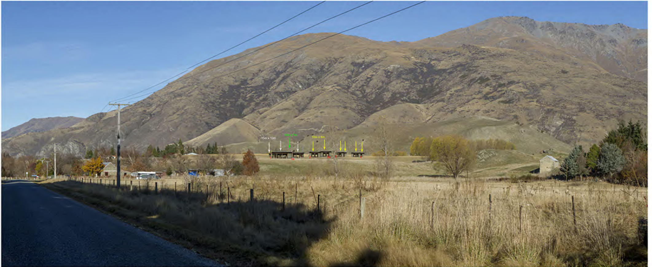
Photo 2b: Potential Buildings - x3 at 15m x 10m (150m); x6 duplex accom units at 10m x 8m (80); x1 10m x 7m (70m). Buildings placed behind each other minimise visibility from Morven Ferry road, while maximising view shafts through to Coronet Peak (North-West)
