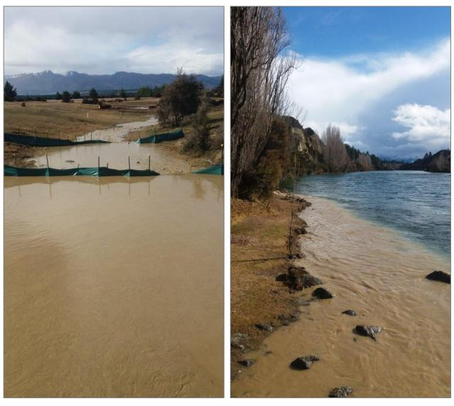
Figure 3: Outlet Road overland flow path and silt fence failure with sediment discharge to the Clutha River
