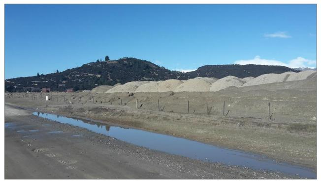
Figure 1: Topsoil stockpiles with no sediment control
