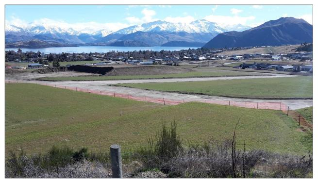
Figure 5: Unstabilised topsoil stockpile
