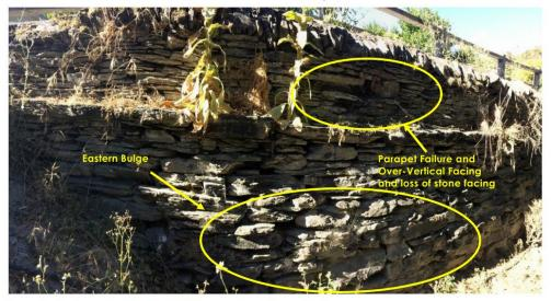
Figure 3 - Photograph of Eastern Wall Segment and Parapet Failure
