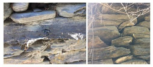
Figure 4 - Stones Cracking in Facing Near Eastern Bulge
