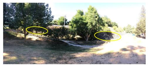
Figure 2 – The Retaining Wall viewed from Butlers Green, bulging areas marked in yellow
