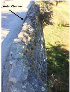
Figure 8 - Western Wall Failure From Above
