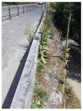
Figure 6 - Parapet and Wall Deflection As Seen From Above
