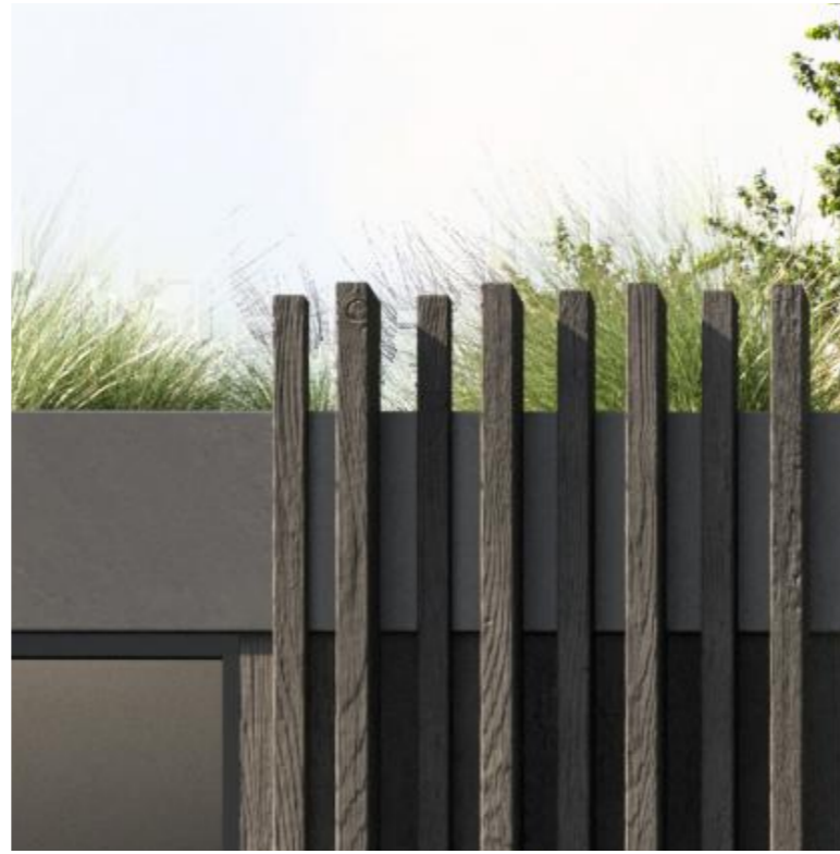
Cladding: rough-sawn timber extends above green roof edge, to provide a soft edge All flashings, fascia and barge boards to be matt and have an LRV of <30%
