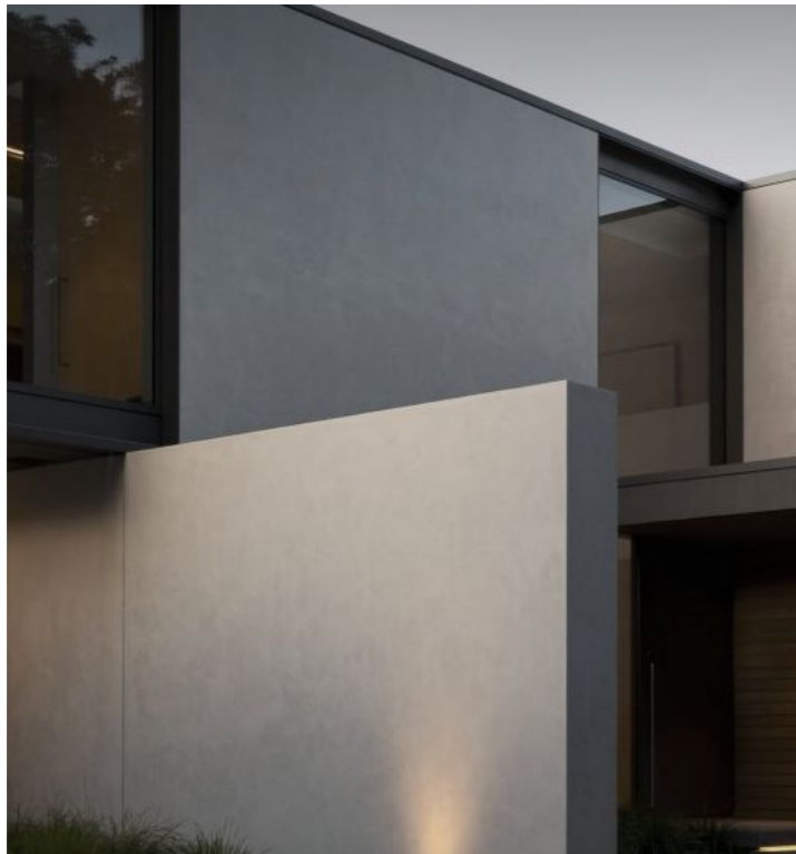
Tanking walls: Precast concrete, or plastered walls with a mid-tone grey concrete finish having an LRV of <30%
