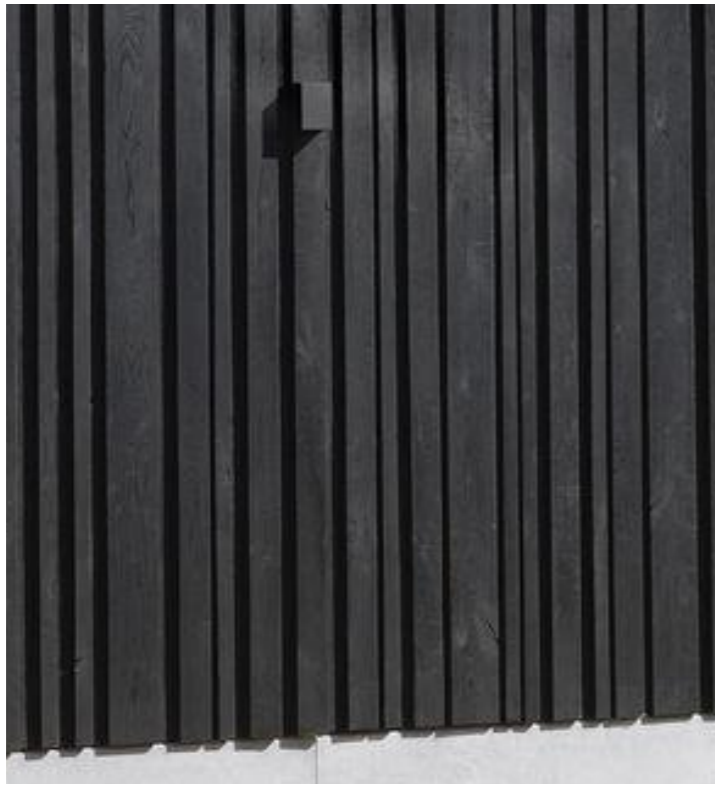
Cladding: rough-sawn timber over plywood, with random spacing and depth Resene Nero exterior wood stain or similar. LRV <30%
