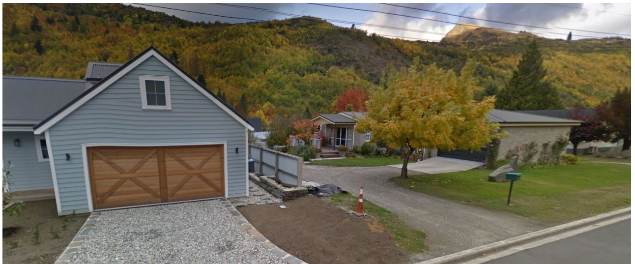
Figure 3: Garages located at 33A and 35 Devon Street
