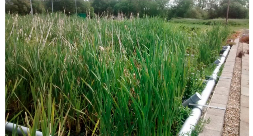
Example: Petersfield WWTW Tertiary Subsurface Wetland (UK), 10 x 1600m 2
