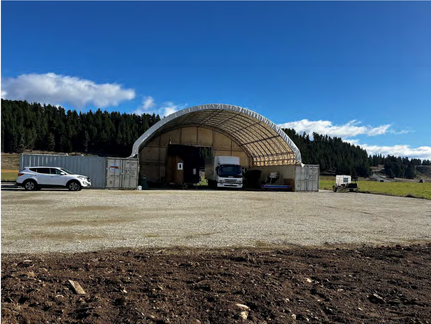
Figure 4 The existing building
