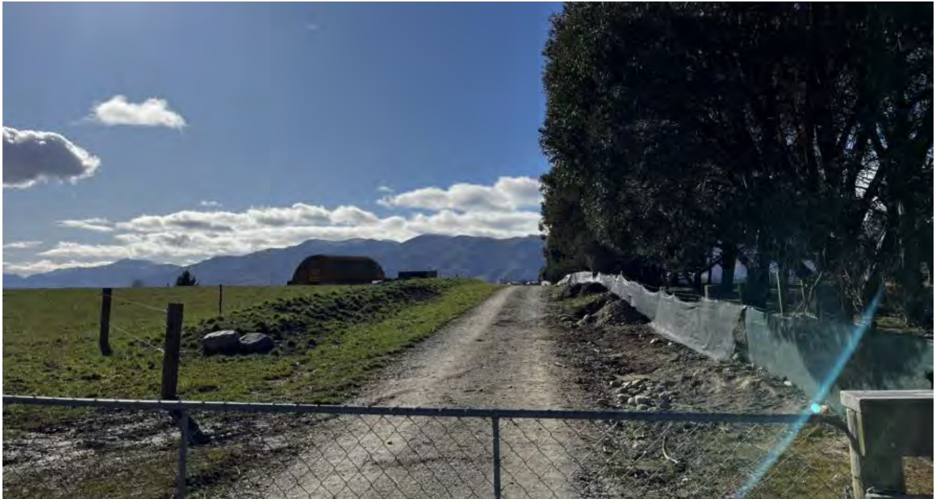
Figure 12b Showing the existing building re-coloured as viewed from SH6 vehicle entry point
