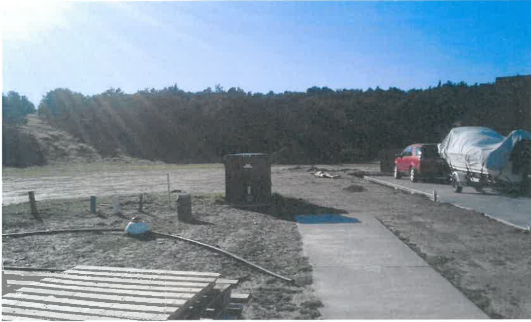
Image 23 – 1.0m wide walking track connection point
