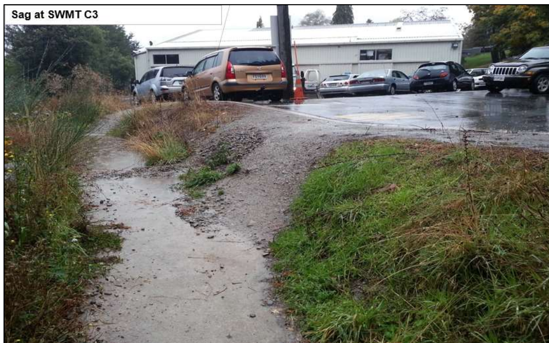
Figure 4.3: Sag Point at SWMT C3
